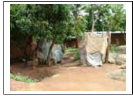
Two typical toilets
