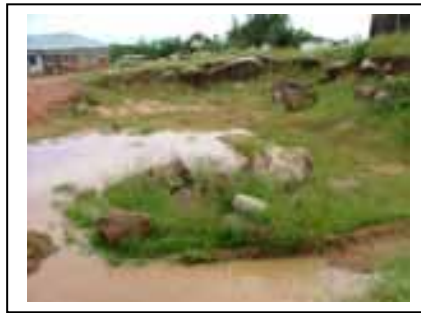
Standing water near the dispensary
