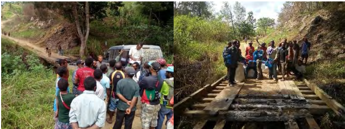
Fig.10 – Distributions At Broken Bridge In Movi
